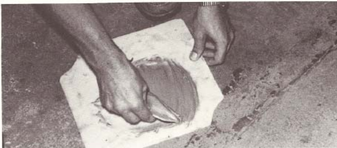
Step 4. Mix the body filler and cream hardener according to the directions
